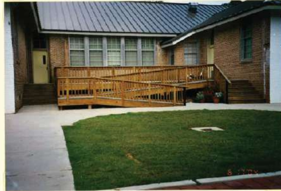
Dixie Attendance Center Back of Main Building Changes made - 2002-2003
