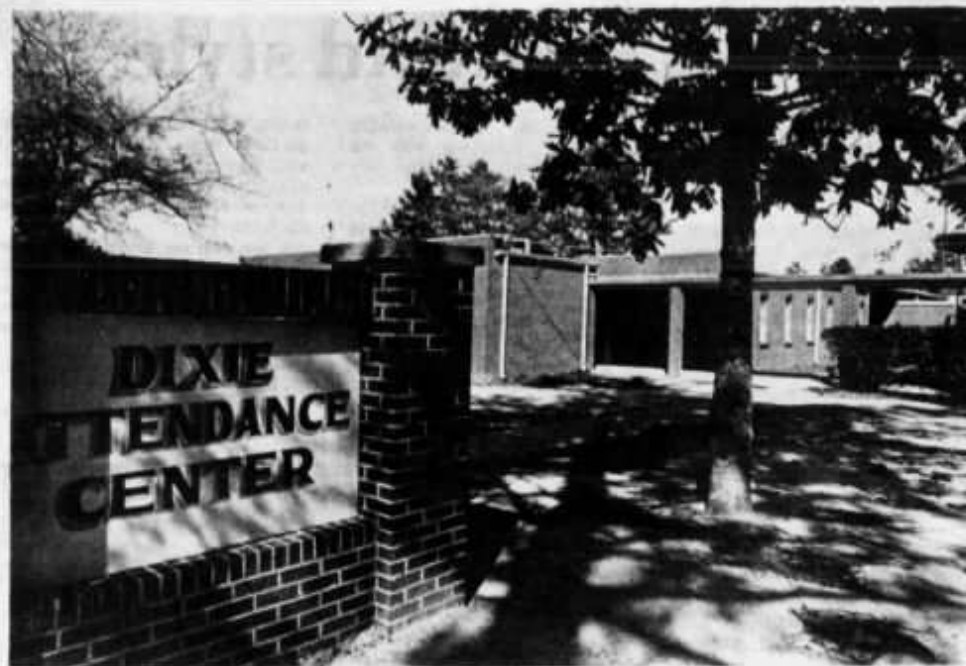
Four new classrooms, a principal's office and a teacher workshop were among the facilities completed at Dixie Attendance Center in February, 1979. Cost of the project was approximately $126,000. The addition adjoins the old Dixie building, which was constructed in 1921.
