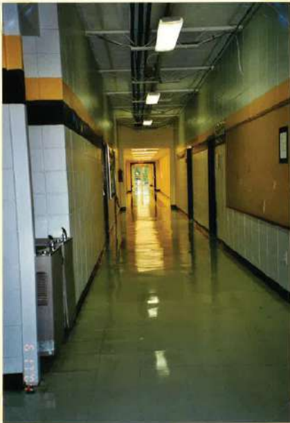
Dixie Attendance Center Office Building View from office down hall by existing and new classrooms Changes made 2002-2003
