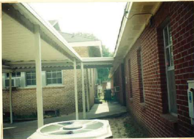
MAIN BUILDING Southwest Corner Picture made June, 2000
