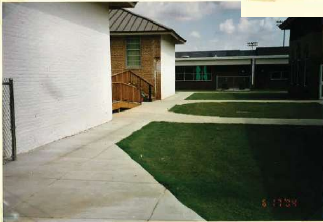
Dixie Attendance Center White walls - location of old bathrooms that had been added to the Main Building in the past Picture was made facing the North Changes made - 2002-2003
